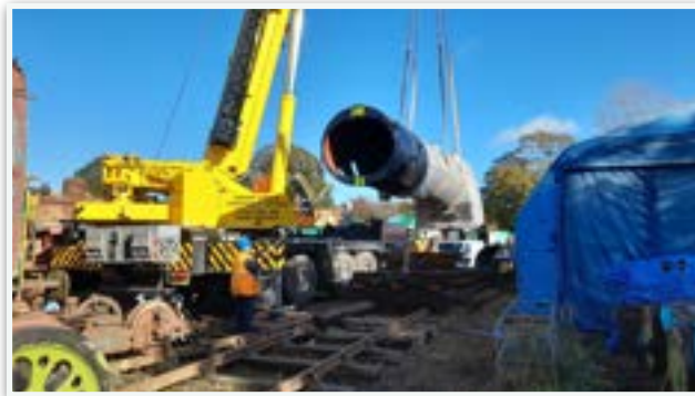
The boiler lift
